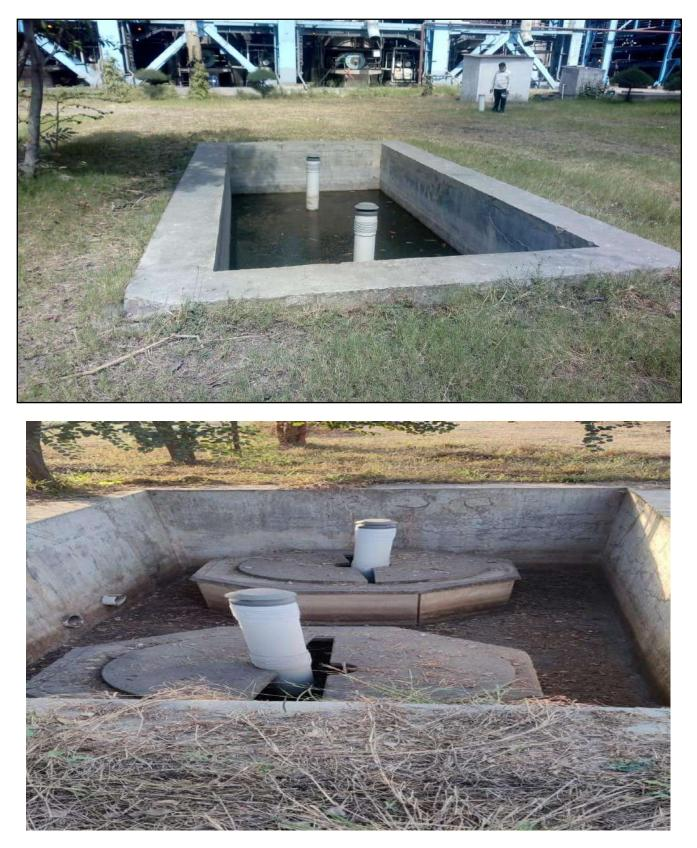
Fig 7.1: Rain water Harvesting in the plant premises
